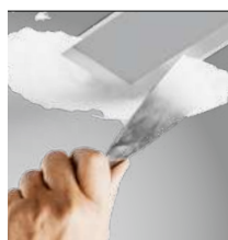
skimmed into plasterboard ceiling (trimless)
